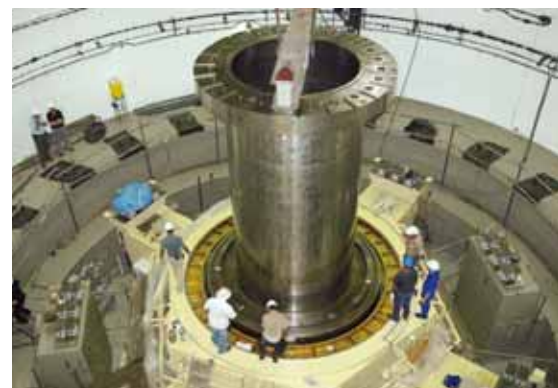
Installation of the generator shaft
