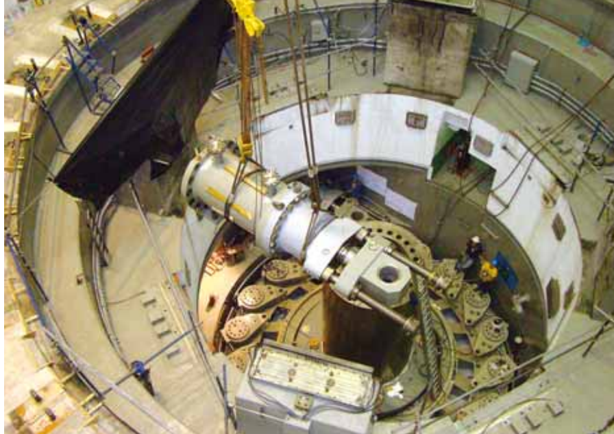
Re-assembly of the servo motor
