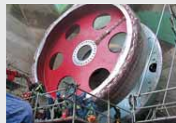
Generator rotor installation
