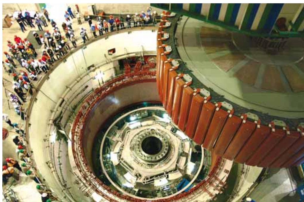
Installation of generator rotor
