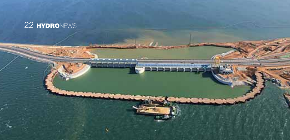
Construction site flooded before coffer dam removal
