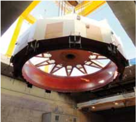
Bemposta stator lifting into pit
