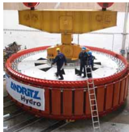
Generator rotor ready for lifting into final position
