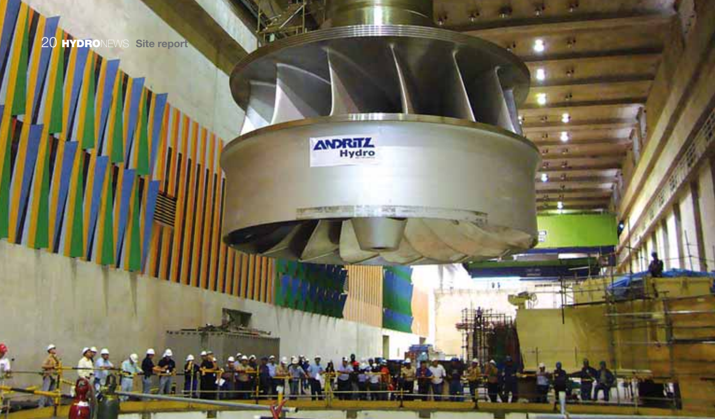
Installation of turbine runner
